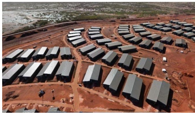
500 resort-style rooms installed at Kens Bore
