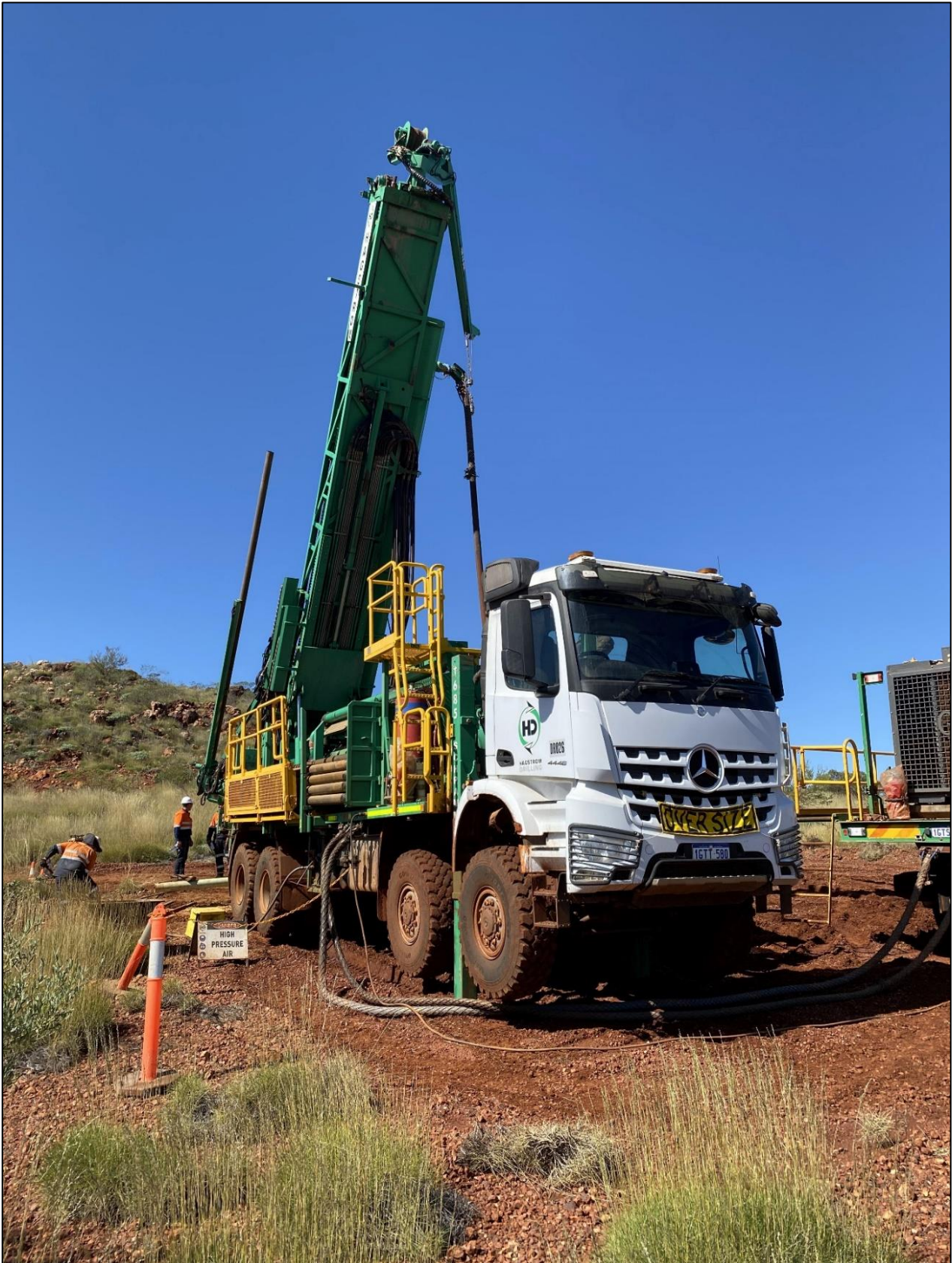
Figure 2 - RC Drilling for Red Hill at the Dereks Bore Gold Target. DKRC0001 was drilled at 60° angled to the east (90° azimuth). EOH 348m BGL.
